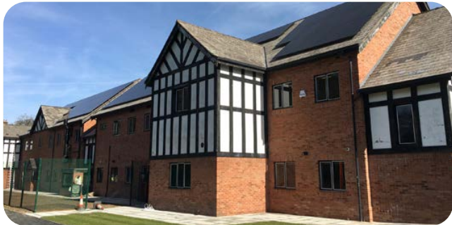
Cheshire Hall School Solar panels installed
